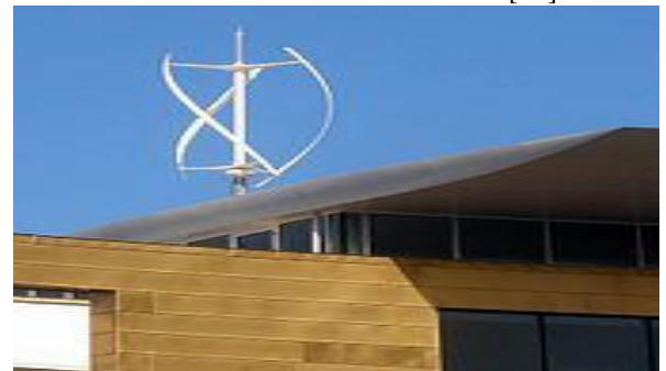
Figure 6. A 6.5 kW rated Gorlov type VAWT, with a height of 5 m and diameter 3m in Bristol [21].
