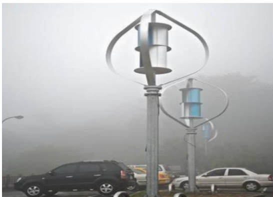
Figure 8b. Hybrid VAWT generator (Darrieus and Savonius) [32]
