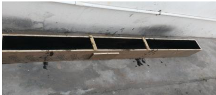
Fig. 5 Wooden Beam Mould
