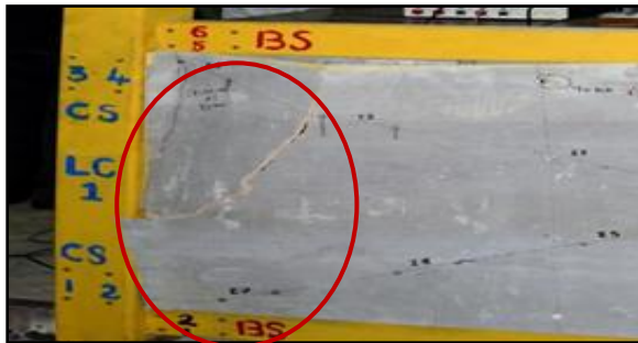
Fig.31 Crushing of Infill at Compression Corner-Frame (2)
